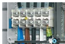
Terminals for incoming/outgoing cables under accessories
