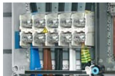
Terminals for incoming/outgoing cables under accessories
