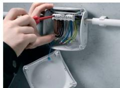
retaining strap prevents the lid from falling or losing and makes daily installation work easier
